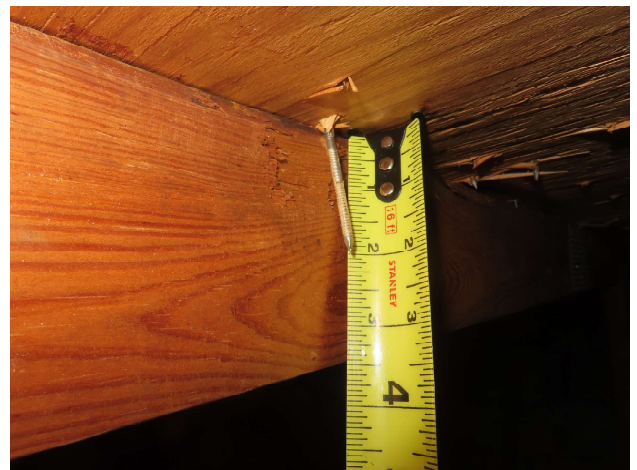
Roof deck attachment - 8d nails
