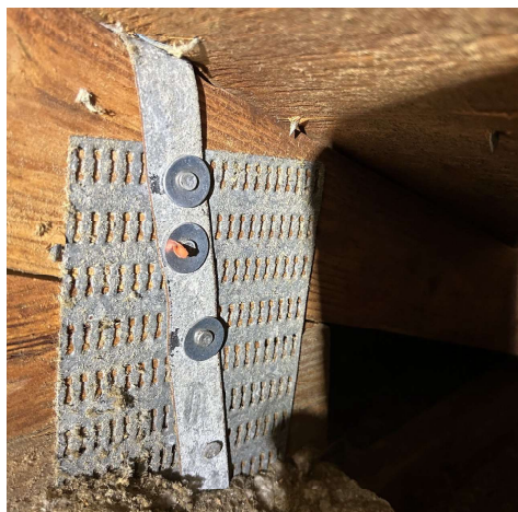
Roof to wall attachment - Clips
