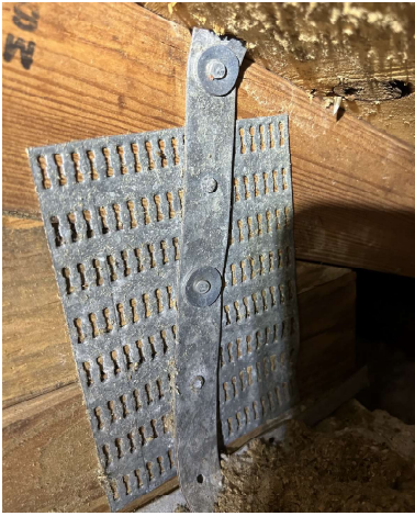
Roof to wall attachment - Clips
