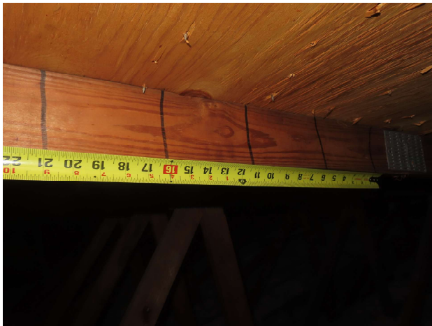
Roof deck nail spacing - Field
