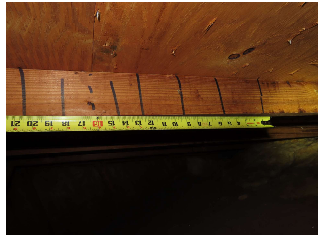
Roof deck nail spacing - Edge
