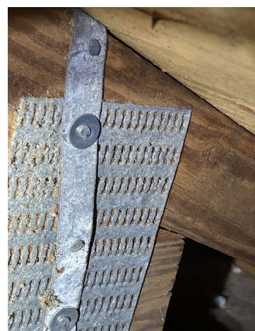
Roof to wall attachment - Clips
