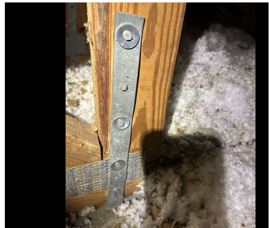
Roof to wall attachment - Clips
